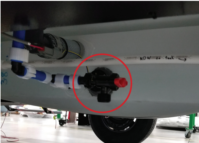
Fresh water tank drain valve circled in red
