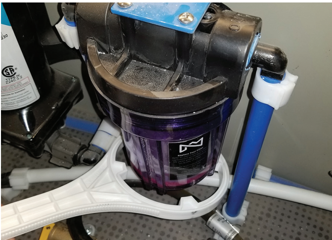
Use filter wrench, slide up from underneath
