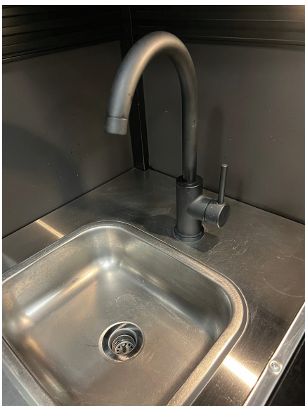
Stainless steel sink in kitchen
