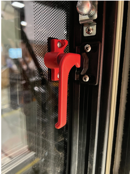
Proper position for window latches
