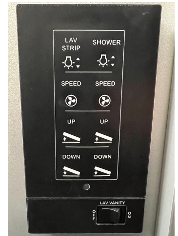
Bathroom wireless switch panel
