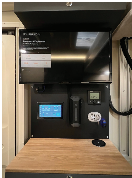
Entertainment cabinet control panel
