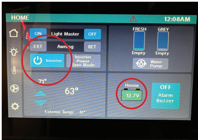
Turn inverter on at touch panel screen, check battery voltage level
