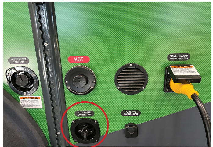
Fresh city water connection circled in red
