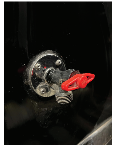
Outside hose spigot located behind front storage box, street side
