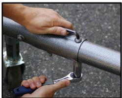
**Step 8**: Insert M12 bolts. Flat washer and Hex Nut are installed from below. Tighten to 40 ft-lb (54 Nm).
